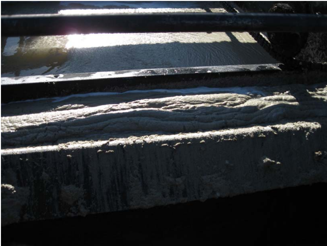
DAF skimming sludge off of the Treated Water
